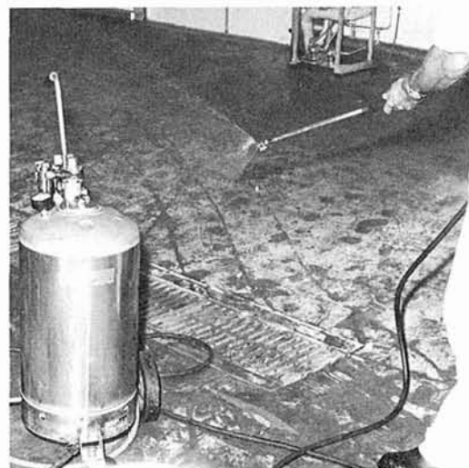
Fig. 4. Gel cleaning.
