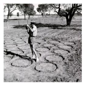
Most tiresome. Similar readings were taken on some other occasions from gypsum blocks buried at varying depths. These readings gave soil moisture information. The gypsum blocks were connected by cables to switches, which in turn were plugged into a wheatstone bridge or resistance box (or simply, R-box). You sat inside a small shelter made of compressed straw panels to operate the R-box.
